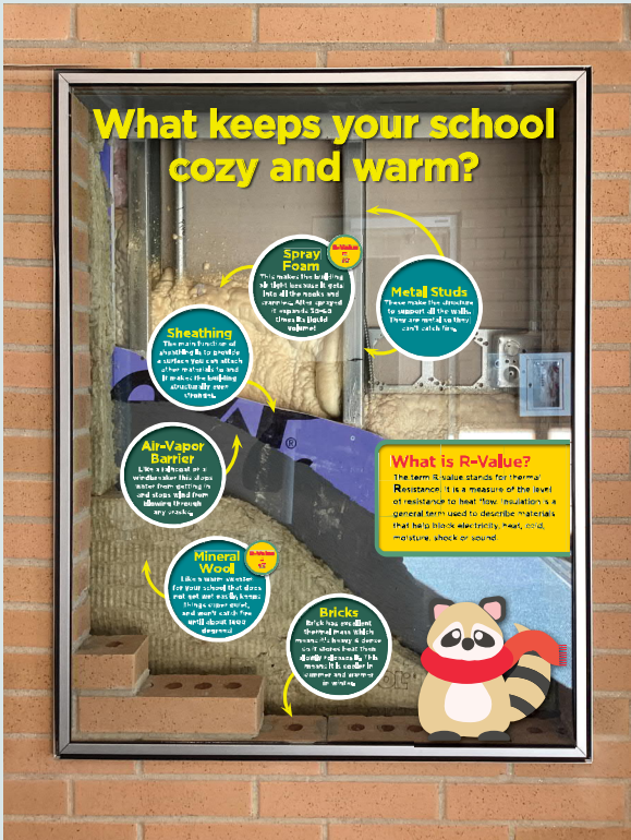
A custom-graphic at the school entry reveals a cut-out of the wall assembly of the school, helping students see what is inside the walls that surround them, and how each of the materials play their own part in the assembly.
