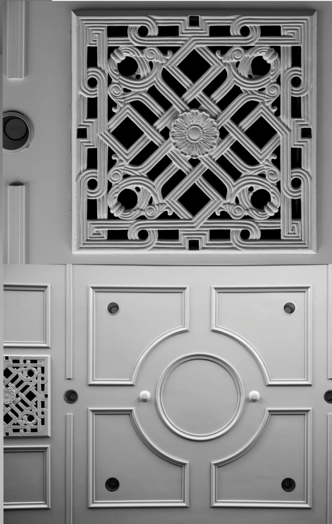
Replicated Historic Auditorium Ceiling Details, Including GFRG Corbels, Mechanical Grilles, and Patterned Trim Molding.
