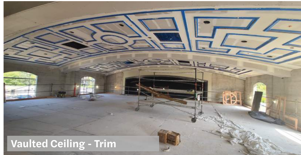
Vaulted Ceiling - Drywall Finish
