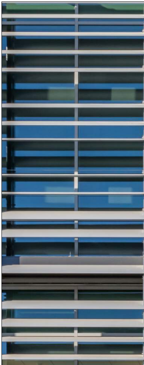
Aluminum Curtain Wall with Low-E Glazing and Aluminum Airfoil Shading System
