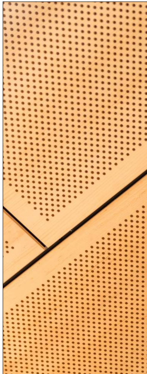
Staggered Acoustical Wood Ceiling Panels
