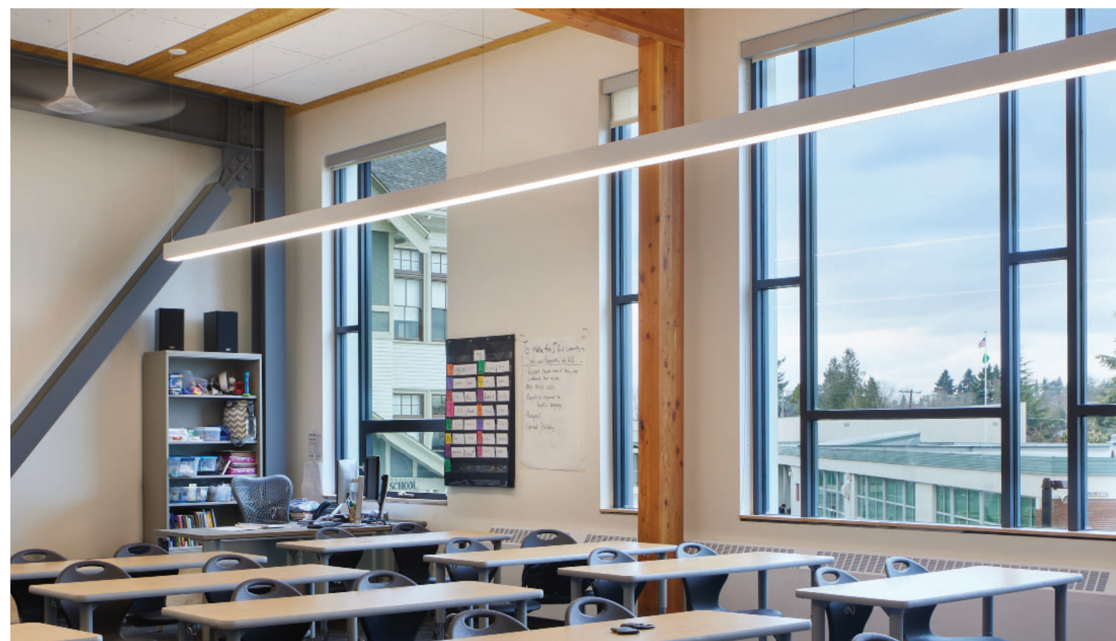
The top image shows the restored 1909 classroom with views of the new CLT classroom addition. The bottom image shows the new classroom with CLT ceilings and views of the restored schoolhouse.
