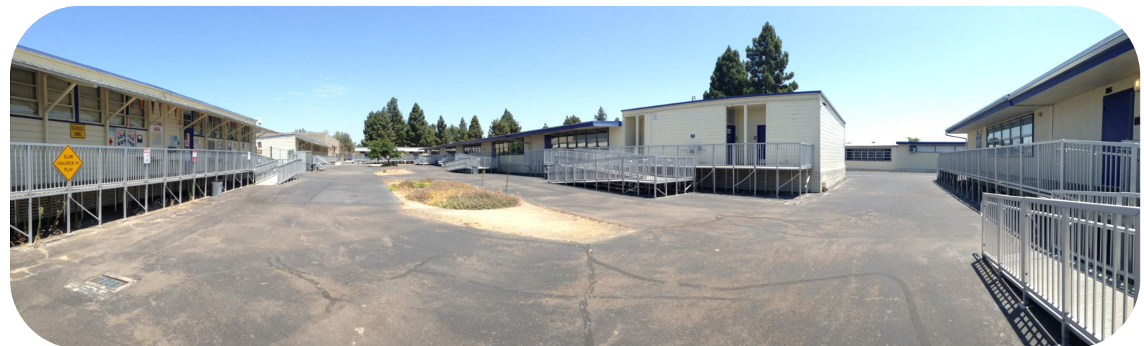
PORTABLES TO BE REPLACED
