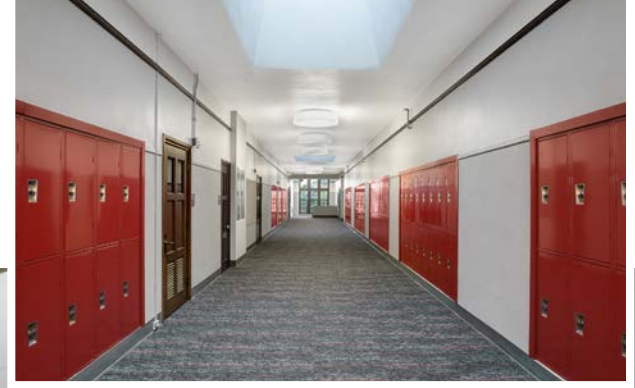
RENOVATED HALLWAY WITH ADDED DAYLIGHTING
