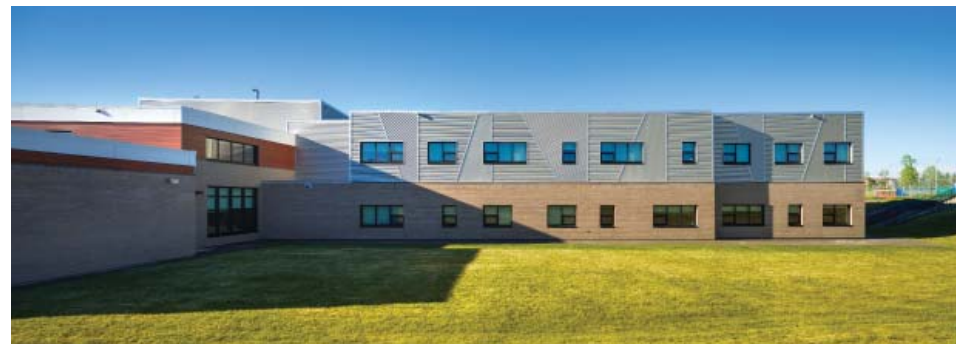
Above: The top image faces the corner of the brownfield site (looking southeast) from the perspective of Fish Creek Boulevard. The middle image demonstrates how the school fits within the sloping of the site as well as how the one- and two-storey sections of the school connect. The bottom image shows how the two-storey section of the school offers privacy and protection from the elements in the outdoor play spaces (e.g., playground and field).
