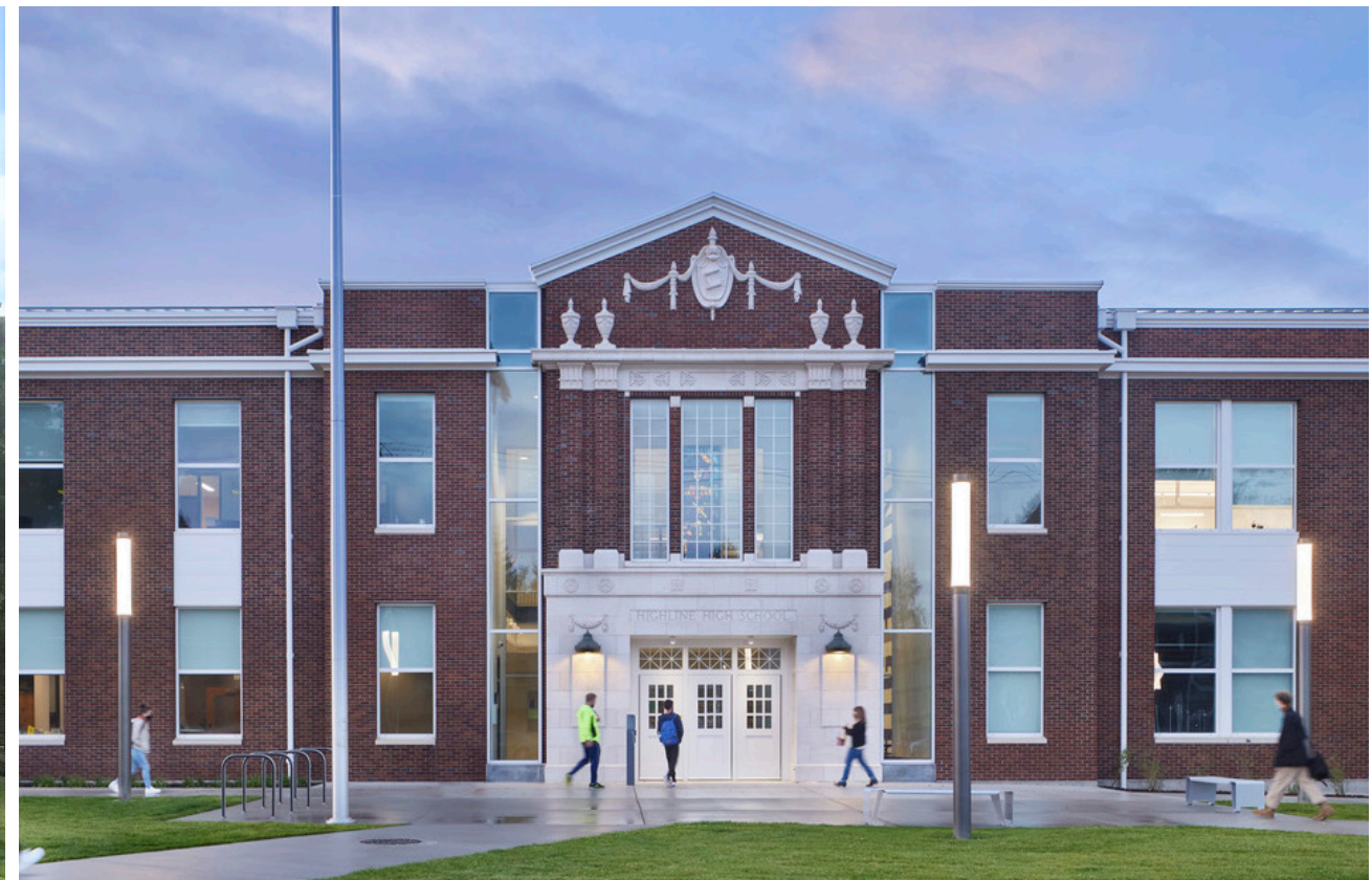
The replacement school retains the look of the original building. Terra cotta was salvaged from the original school and used for the new entry. The original brick was intended to be salvaged but it was discovered they contained asbestos.
