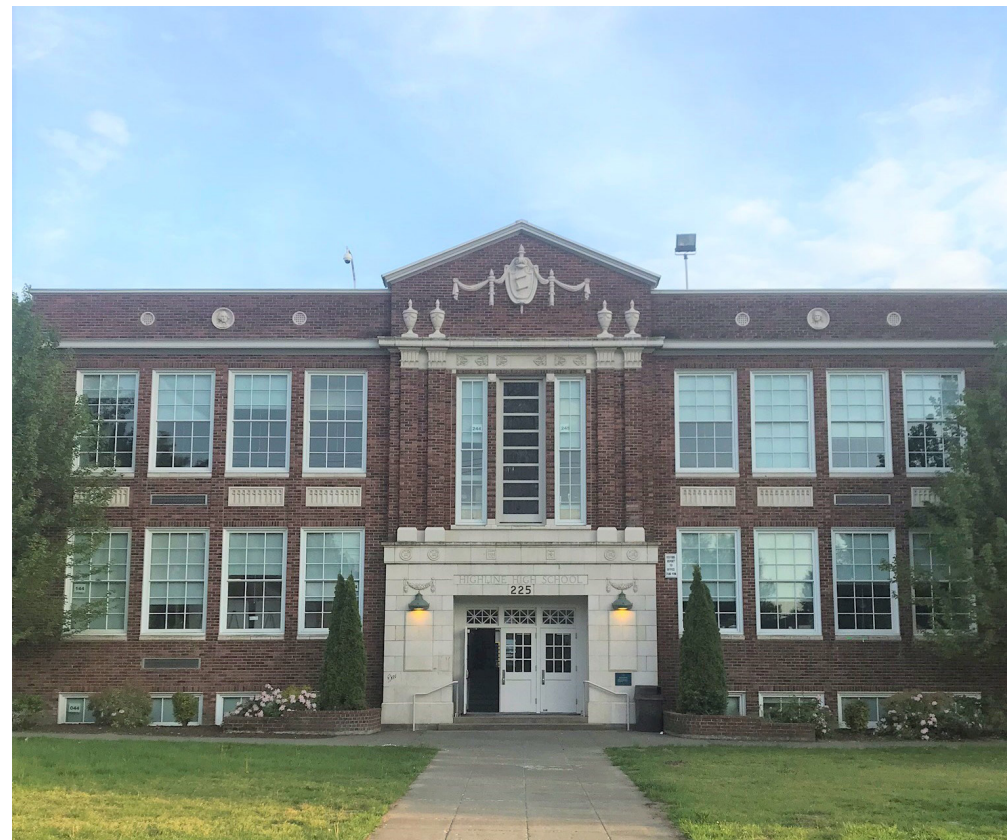
The original Highline High School entry prior to demolition.
