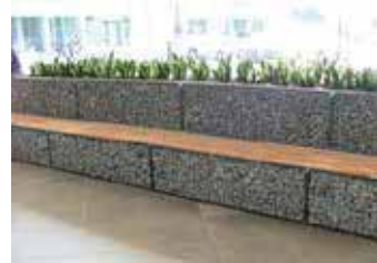
6 Custom Gabion Benches
