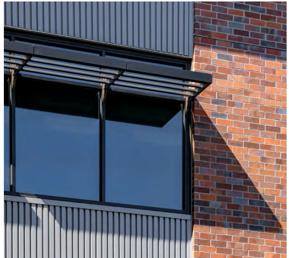
Sunshades block the entry of direct sunlight from the south and reduce overall energy consumption.
