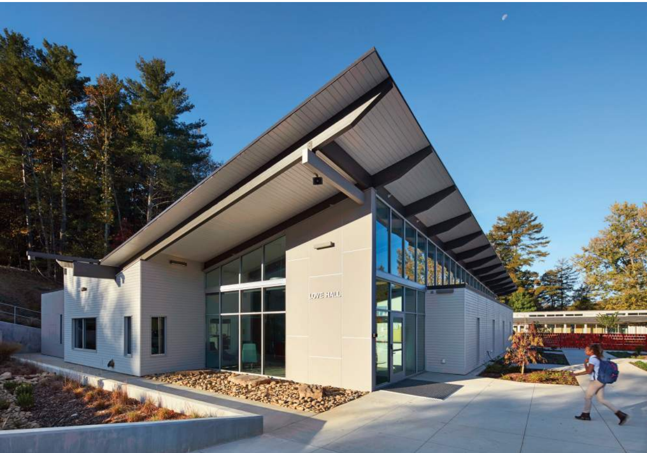
Butterfly roof prominently directs storm-water into rain-garden at entry
