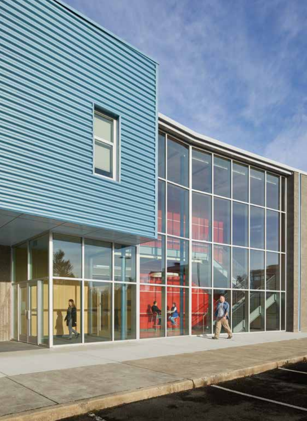
Phase 2: New Academic Building Entry
