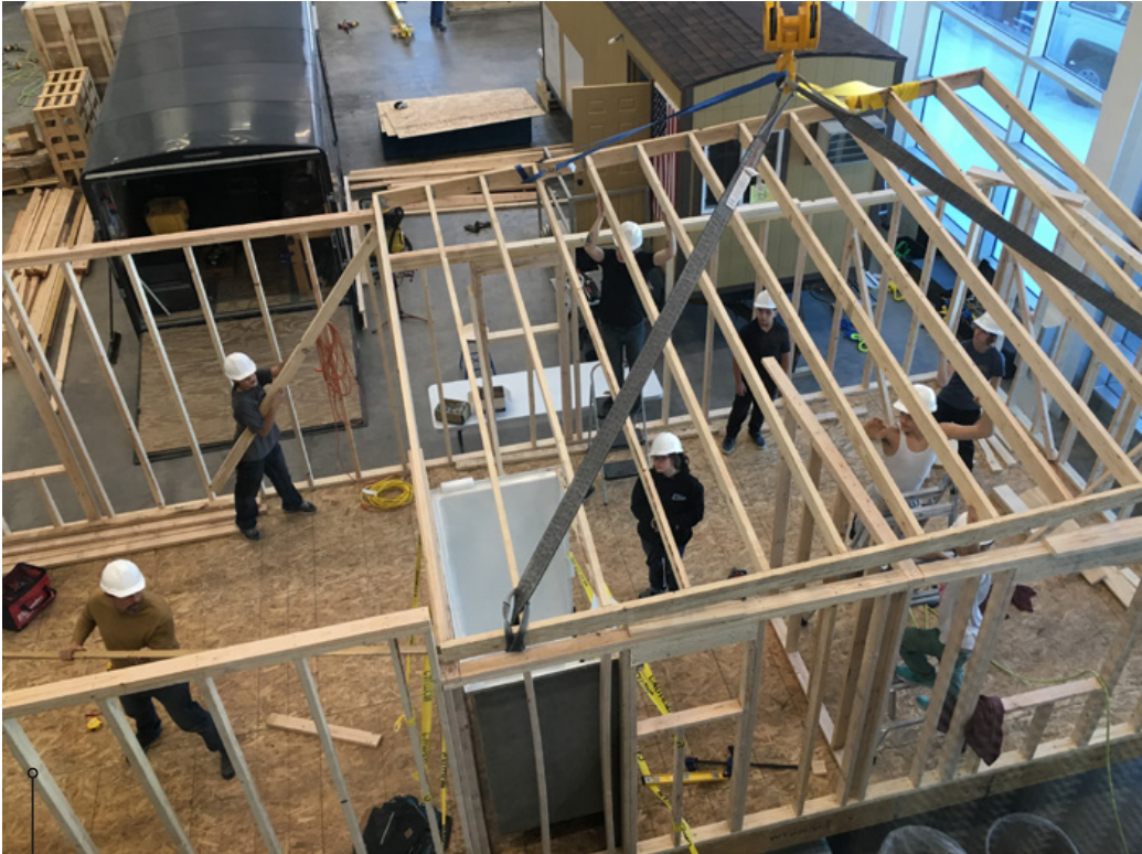
→ Students work together on large-scale projects across academies in the fabrication hall. More than 100 students worked on the construction of a cabin that was auctioned at a community open house.
