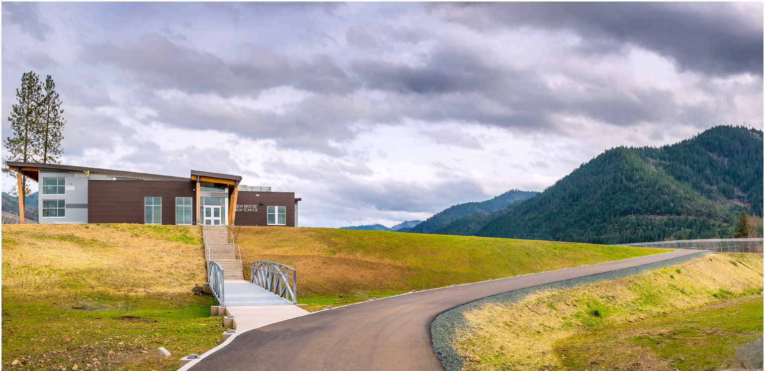
The students' view of New Bridge High School as they approach the bridge from their living units
