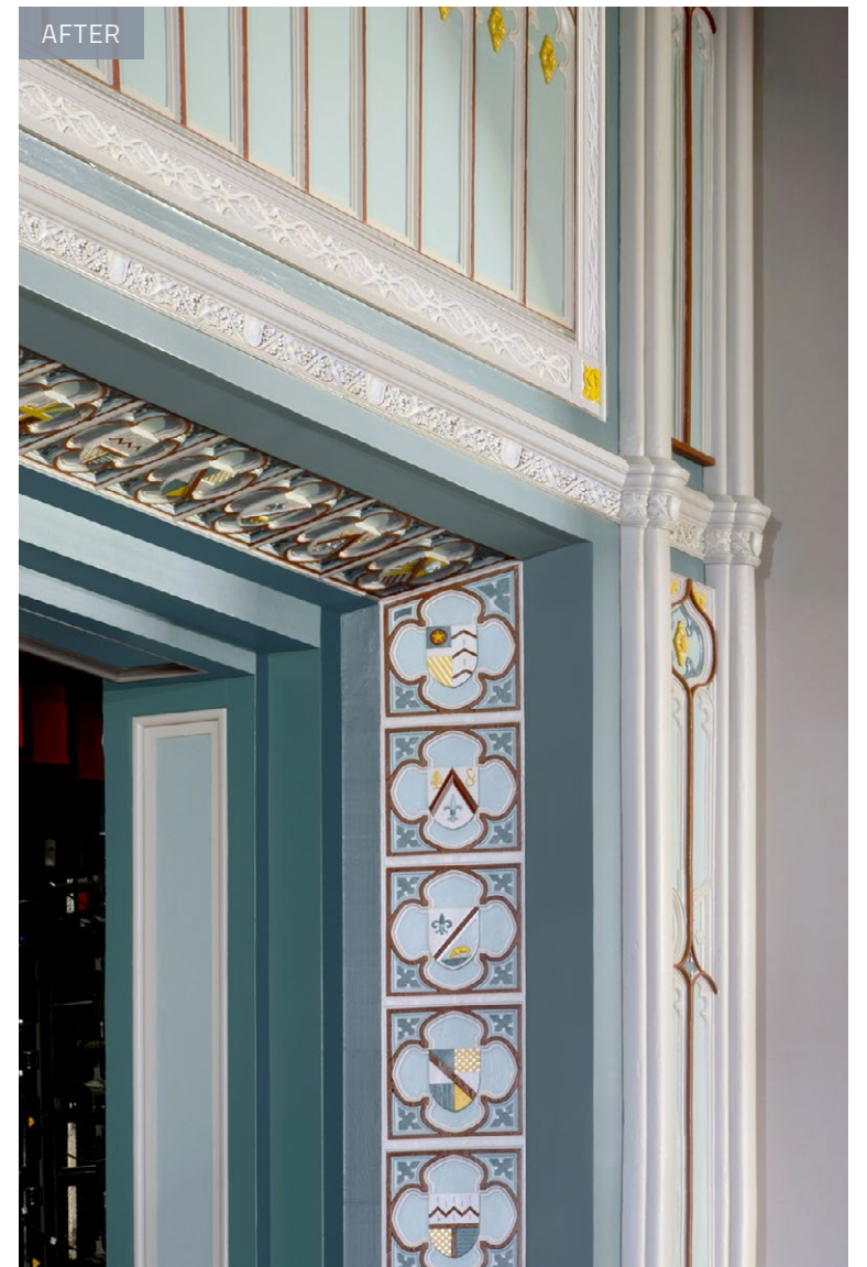
Restored exterior terra cotta and interior decorative plaster.
