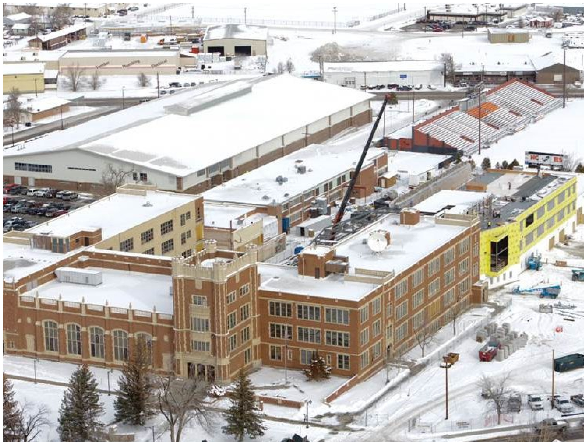
Mid-winter Phase I construction. The historic school is in the foreground and the field house and stadium are in the background.
