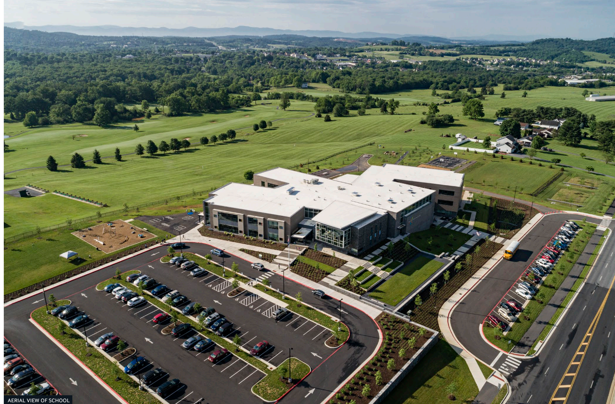
AERIAL VIEW OF SCHOOL
