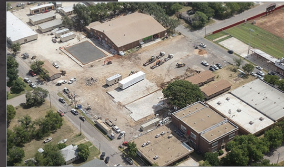
Construction begins on the temporary campus.
