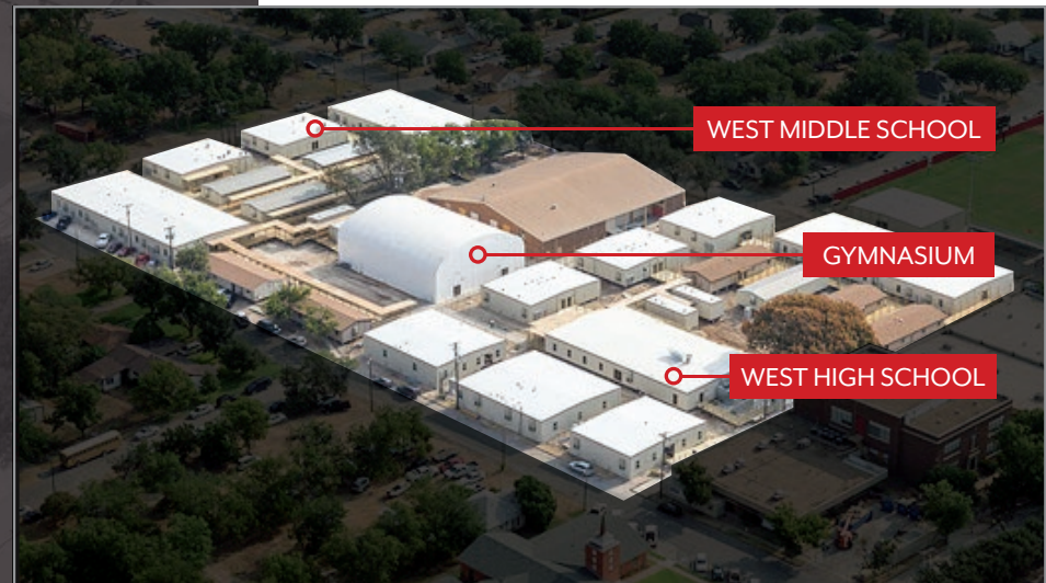
The temporary campus was home to 700 West ISD middle school and high school students for three years. It was constructed on a 6-acre site.
