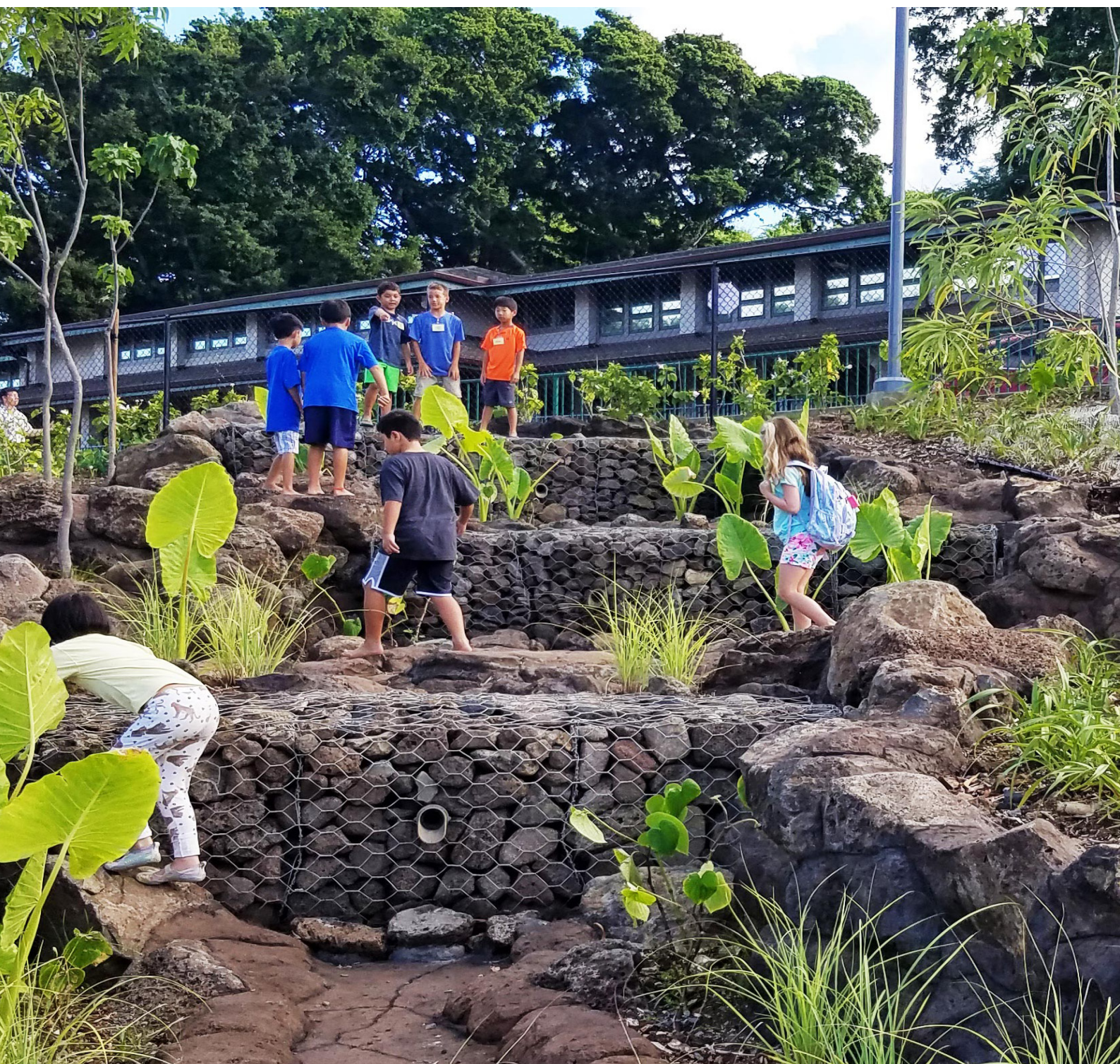
Fig. 2. Rock-lined swale.
