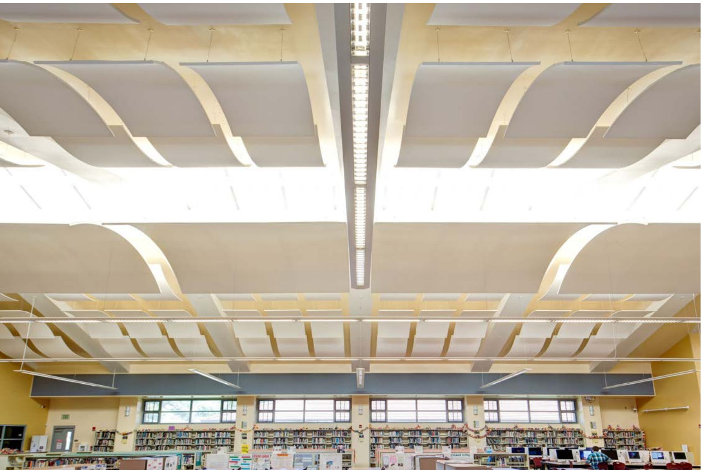
Fig. 5. Main library space with acoustic baffles and clerestory windows.
