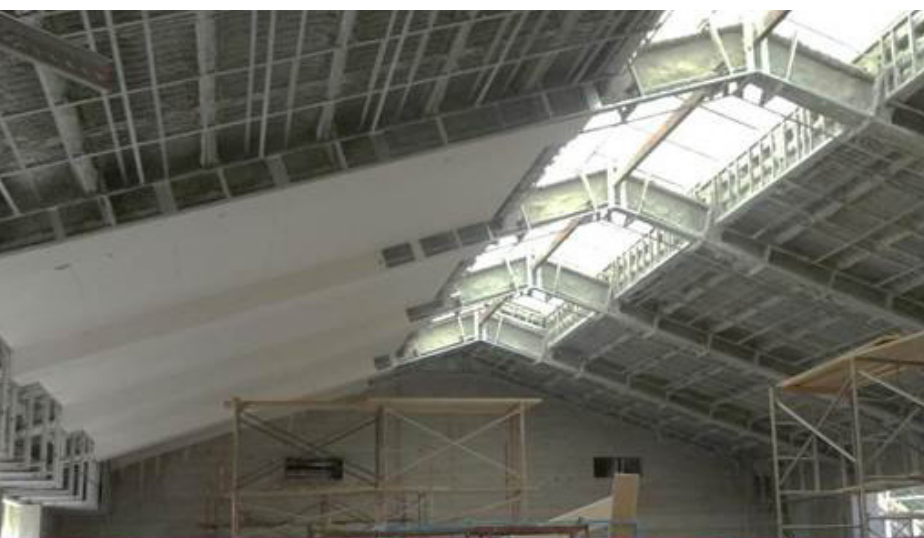
Fig. 11. Skylight and insulated ceiling.
